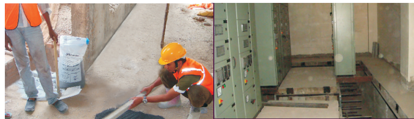
Anti-static flooring in Marconite at RRVPNL 220kVA GIS Sub-station in Jaipur (Rajasthan).
