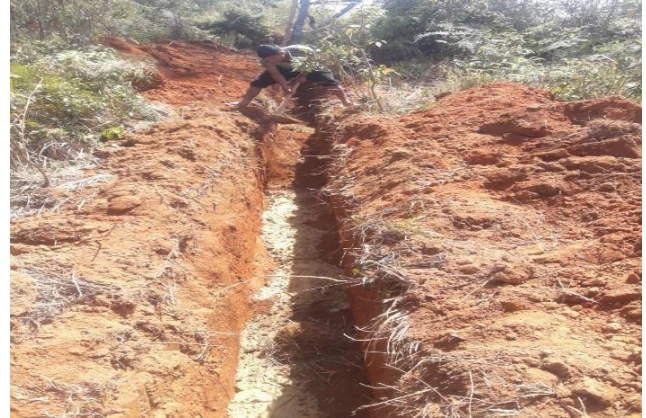
BENTONITE APPLICATION WORK .
