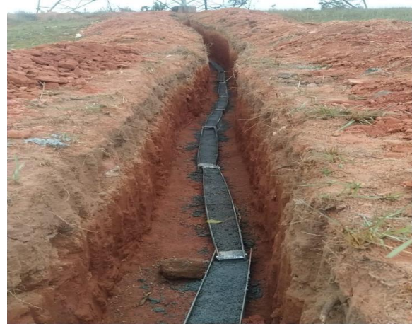
MARCONITE EARTHING EXECUTION WORK
